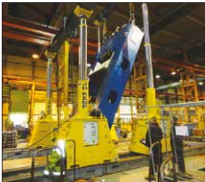
▼ SL400 gantry used to offload and install new forming press.
