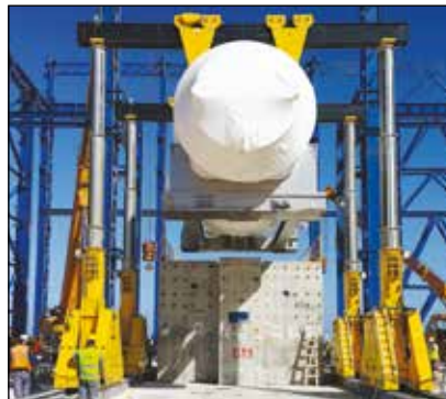
▼ SBL1100 gantry offloading a large generator for installation in a power plant.
