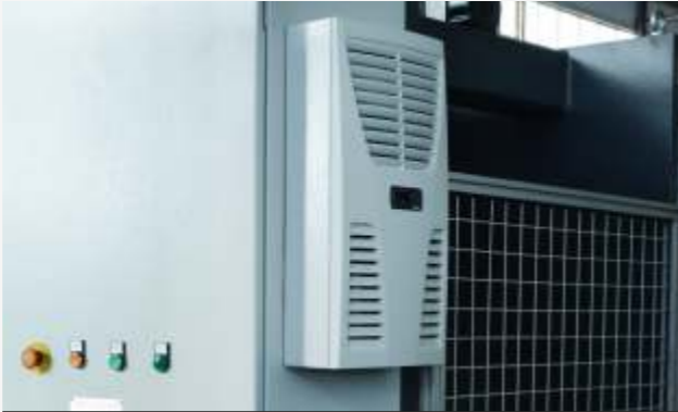
Electrical Cabinet Cooler
