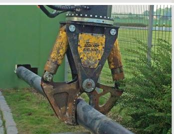
Risk of explosion in an underground cavern storage facility – how can the aboveground pipe system be safely and quickly dismantled? The Darda CC700 S Steel Shear makes this type of work possible.
